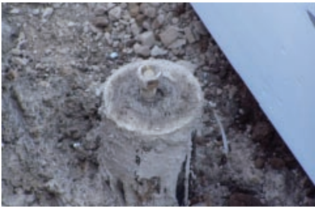
Once the footer crew dug the trench, the piers were cut for the second time. All piers were filled with concrete. Where piers had a final cut at a pipe junction, bolts were installed in the concrete and the bracket was attached to the pier.
