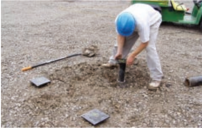
Pre-construction brackets were then placed on each pier. After the installation of the piers, the pad was ready for the remainder of the construction crew to get to work.
