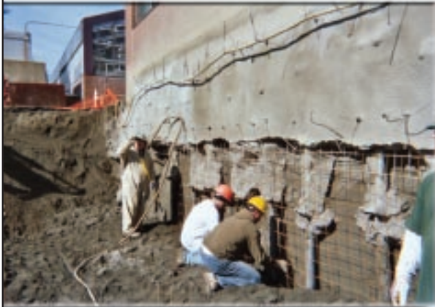
Second row of tie backs installed and being prepared for Shotcrete.
